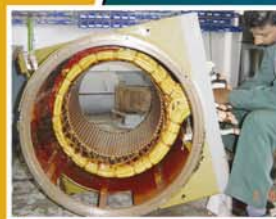
Motor Stator Rewinds
