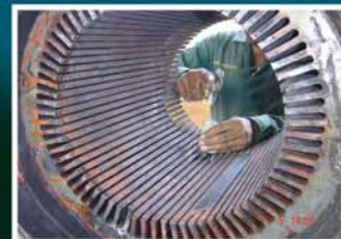
Cleaning of Stator Core
